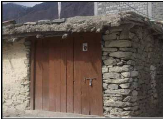
Figure 3: Dry Stone Construction, Himachal Pradesh (Source: Rahul and Ahuja, 2014)
