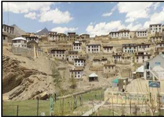
Figure 9: Settlement in Middle Himalayan Region (Source: Kumar and Pushplata, 2013)
