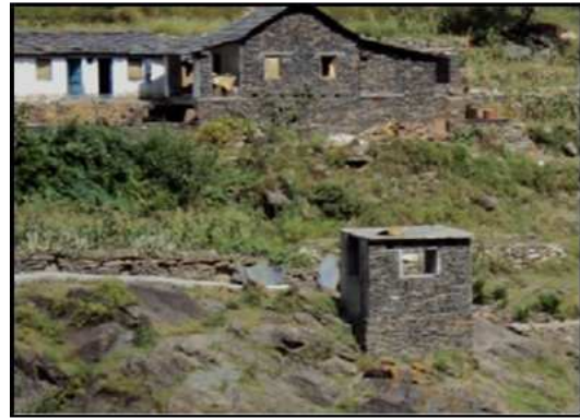
Figure 4: Dry Stone construction, Uttarakhand (Source: Kumar and Pushplata, 2013)
