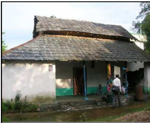
Figure 7: Mud Wall Construction with Sloping Roof (Source: Kumar and Pushplata, 2013)
